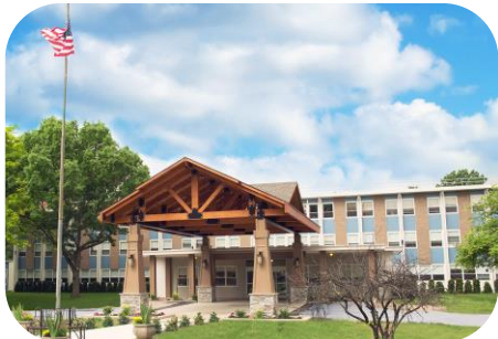
SKILLED NURSING FACILITY Gates, New York Original Assessment $3,306,202 Revised Assessment $1,241,137 Reduction of 62%
