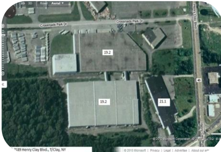
REGIONAL DISTRIBUTION FACILITY Clay, New York Original Assessment $11,154,023 Revised Assessment $7,843,057 Reduction of 30%
