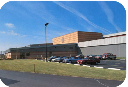
INDUSTRIAL BUILDING Tonawanda, New York Original Assessment $4,608,155 Revised Assessment $3,986,990 Reduction of 13%
