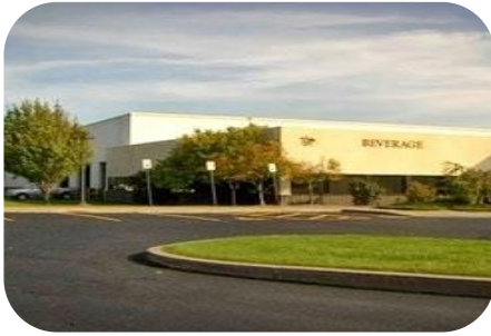
BEVERAGE DISTRIBUTION FACILITY Henrietta, New York Original Assessment $3,328,000 Revised Assessment $2,600,000 Reduction of 22%
