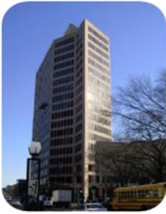
BANK OFFICE New Haven, Connecticut Original Assessment $29,254,610 Revised Assessment $20,500,000 Reduction of 43%
