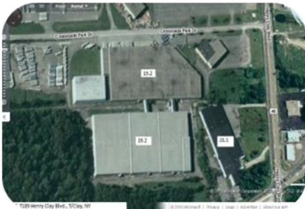
REGIONAL DISTRIBUTION FACILITY Clay, New York Original Assessment $9,945,504 Revised Assessment $7,629,427 Reduction of 23%
