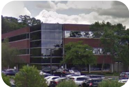
OFFICE BUILDING Perinton, New York Original Assessment $12,202,200 Revised Assessment $4,500,000 Reduction of 63%
