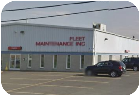
TRUCKING TERMINAL West Seneca, New York Original Assessment $5,160,000 Revised Assessment $2,333,333 Reduction of 55%
